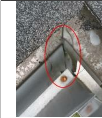
An example of the gutter corner needing sealant maintenance.
