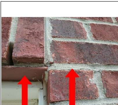
I recommend being diligent with paint maintenance to steel lintels and performing tuckpoint maintenance where cracking exists.
