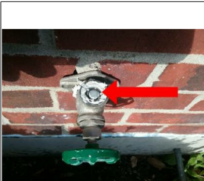
Damaged atmospheric siphon break/cap.
