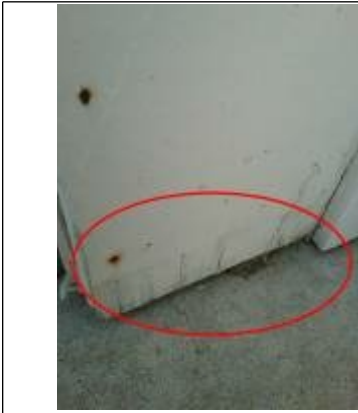
Paint maintenance was needed at overhead door openings.
