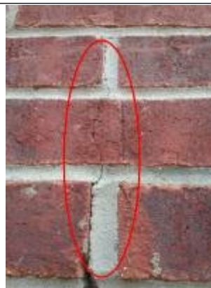
Sealant/tuckpoint maintenance needed and monitor regularly.
