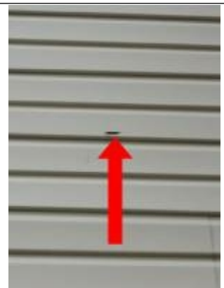
Shown here is a single hole in the siding (East side) that I recommend be repaired.
